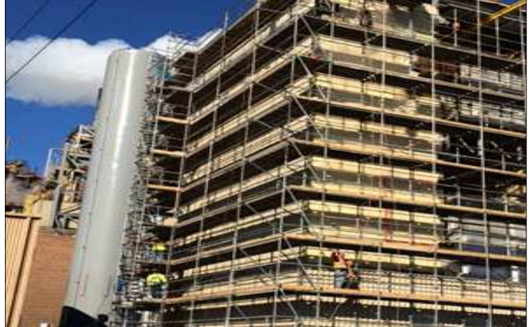
Extensive use of scaffolding for elevated work on bag house project.
