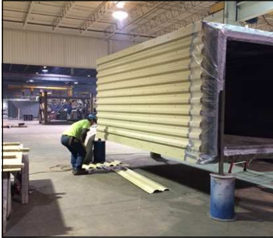
QI employee installing corrugated panels on ductwork.
